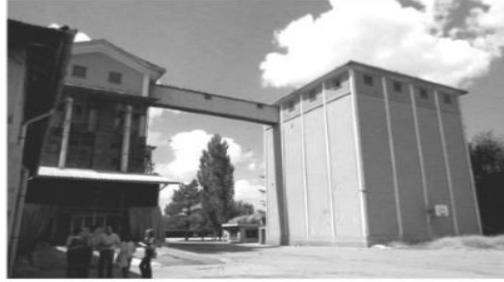
Figure 5. Mühendisler Flour Factory totally demolished in order to erect Özdilek Shopping Mall
