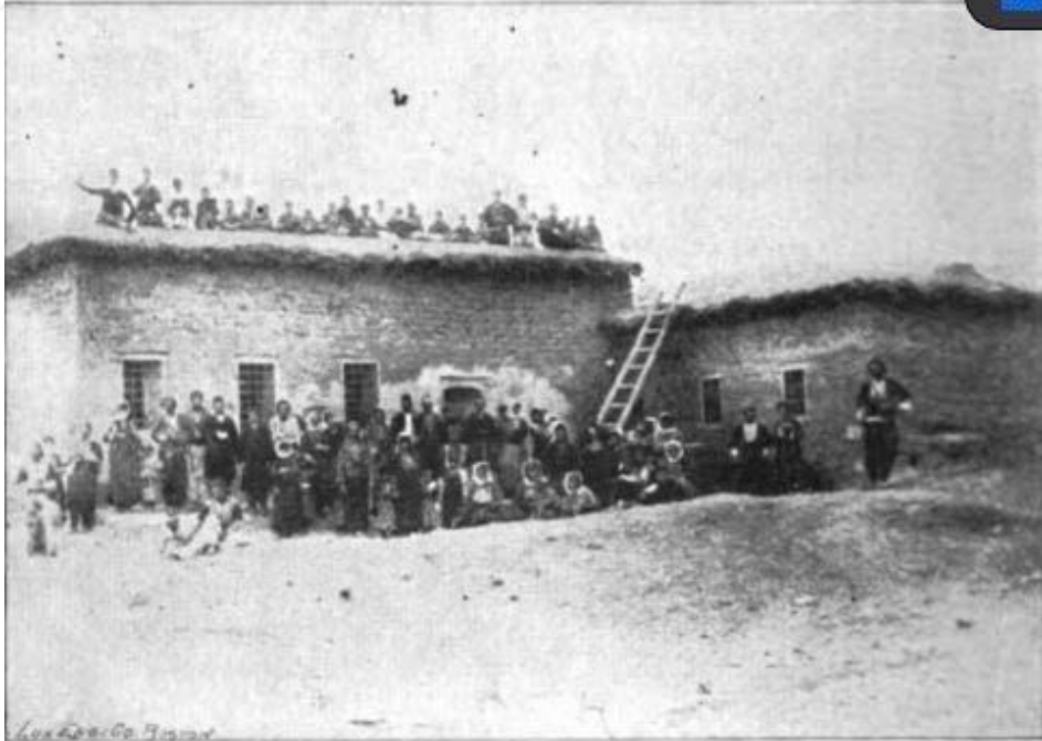
THE CHURCH AND SCHOOLHOUSE AT KALISE,
